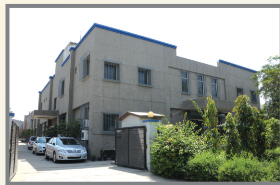
MAIN PRODUCTION UNIT AT GREATER NOIDA
