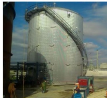
Industrial Storage Tanks
