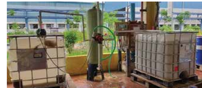
Complete Pilot Plant Installation
